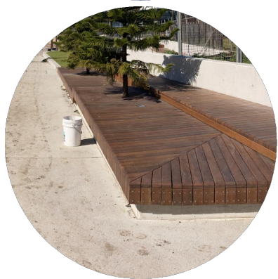
CUSTOM TIMBER SEATING: Concrete base with hardwood timber on top
