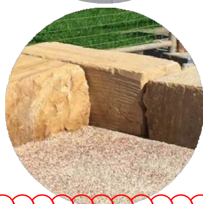
WALL TYPE 2 SANDSTONE LOGS / QUARRY BLOCKS
