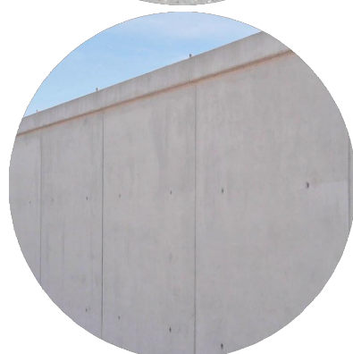
WALL TYPE 1 Insitu concrete walls
