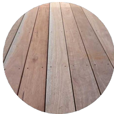
P2: TIMBER DECK TYPE 2 Hardwood timber deck with penetrating oil Surface rating to comply with BCA & ACC & AS
